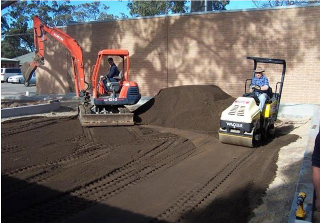
**Figure 5: SPACE structural soil with 100% rootable soil.**
