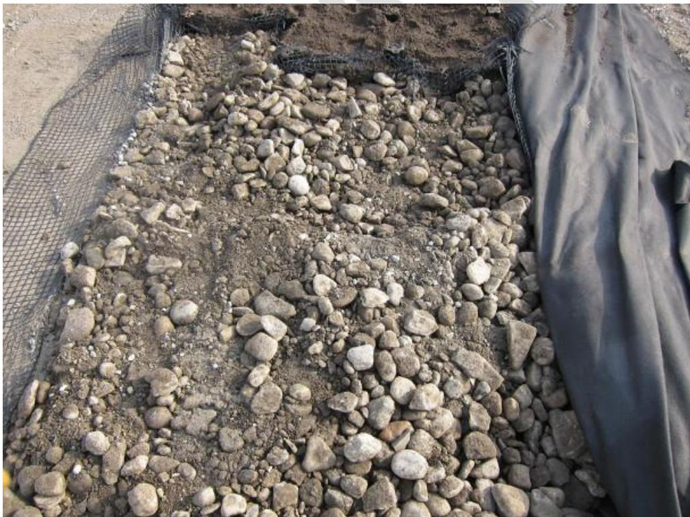
**Figure 4: Stone based structural soil: 80% rock, 20% soil. Source (Urban 2011).**
