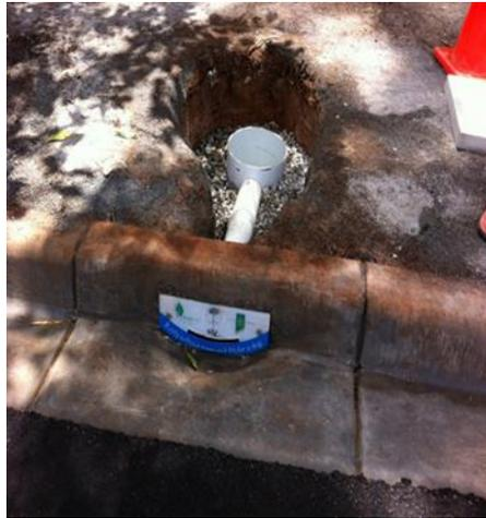
Fig 1: TREENET inlet with leaky well
